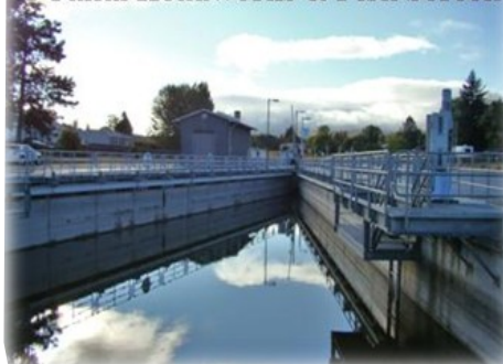
A Canal Headworks & Fish Screen
