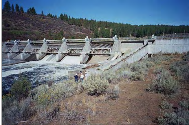
Keno Dam (River Mile 230) is a non-hydroelectric facility and is not part of Reclamation's Klamath Project. The fish ladder facility is visible on the right and is located on the left bank of the Klamath River (looking downstream).
